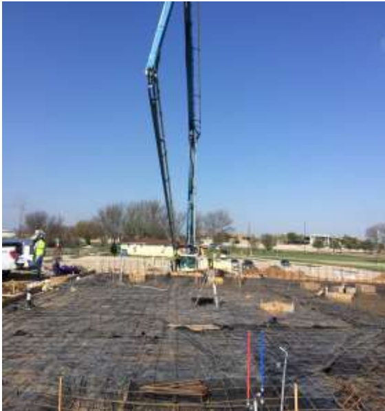
Concrete being poured
