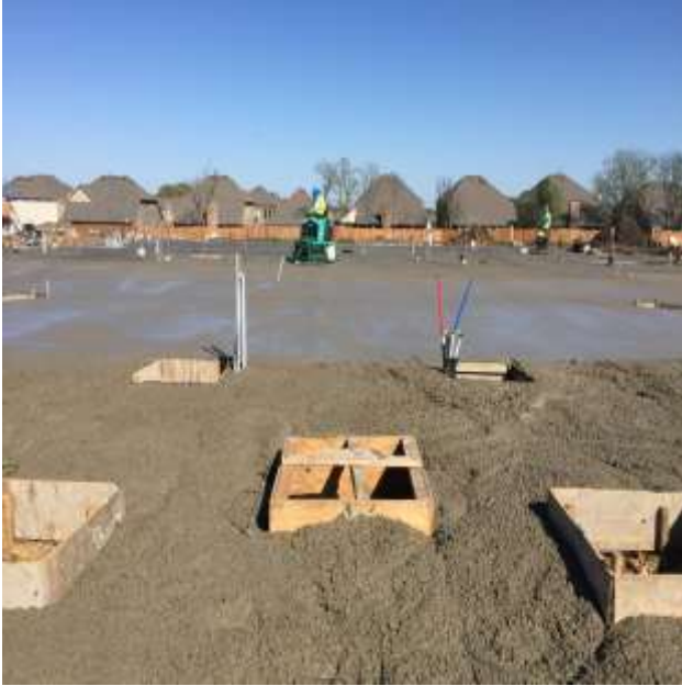
Concrete poured and being leveled
